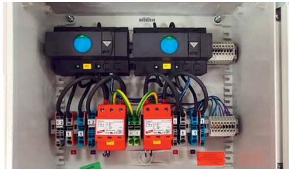
Generator connection box made by enwitec electronic GmbH & Co.KG
